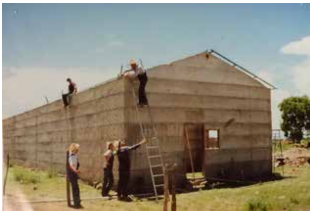
Building a barn
